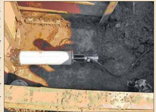
PVC segment and burst head thrust against host pipe by pneumatic clamping device
