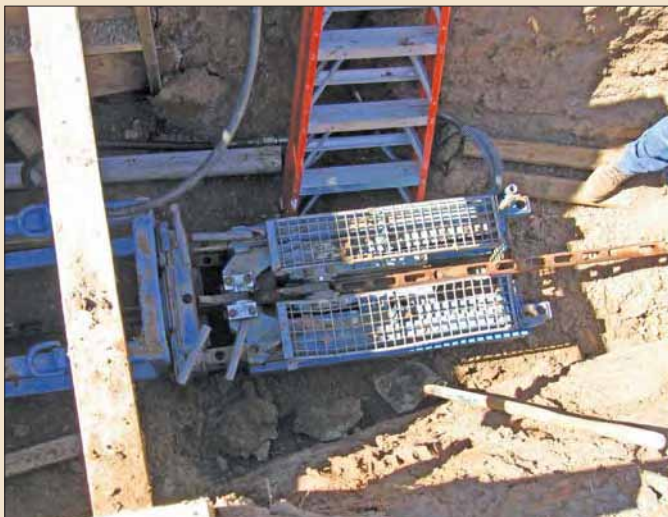
TIP unit in the launching pit during rod pushing operation.
