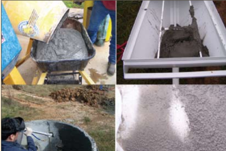
Geopolymer concrete is mixed and sprayed using standard construction equipment.
