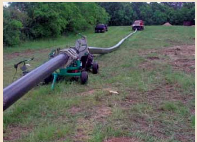
Field testing site at Louisiana Tech South Campus.
